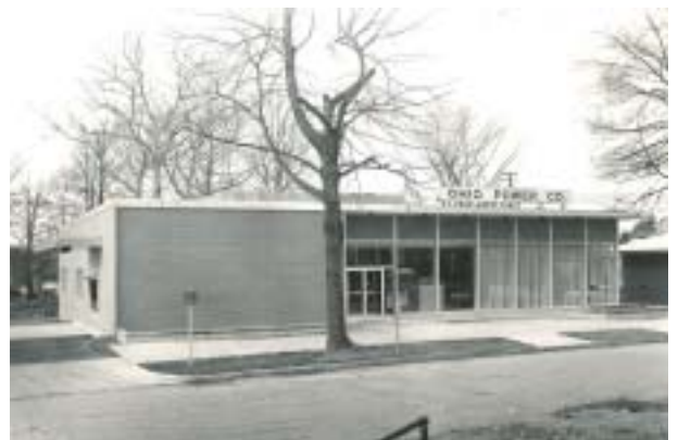
The completed building in 1966
