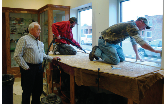
Carl Beynon supervising the repairs in the Education Center
