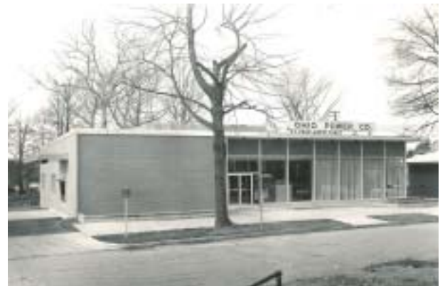
The completed building in 1966
